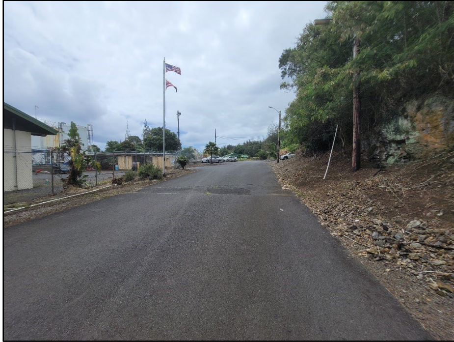
Figure 23. Photo of Kia Manu Street along the mauka side of the plant; view to southeast
