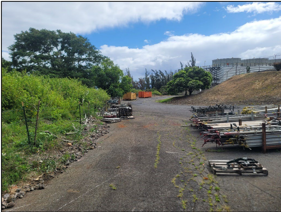
Figure 18. Photo of a staging area at the western edge of the plant, with fuel storage tanks and Kia Manu Street in background; view to northeast
