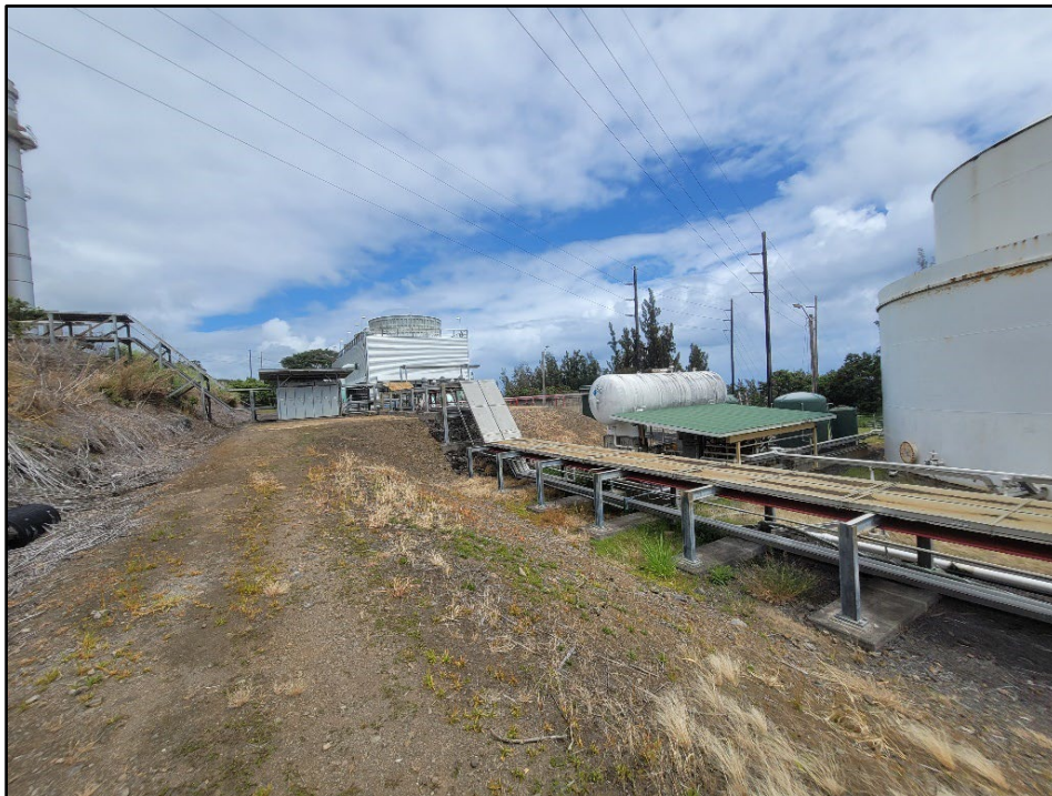
Figure 16. Photo overlooking the central portion of the plant; view to northwest
