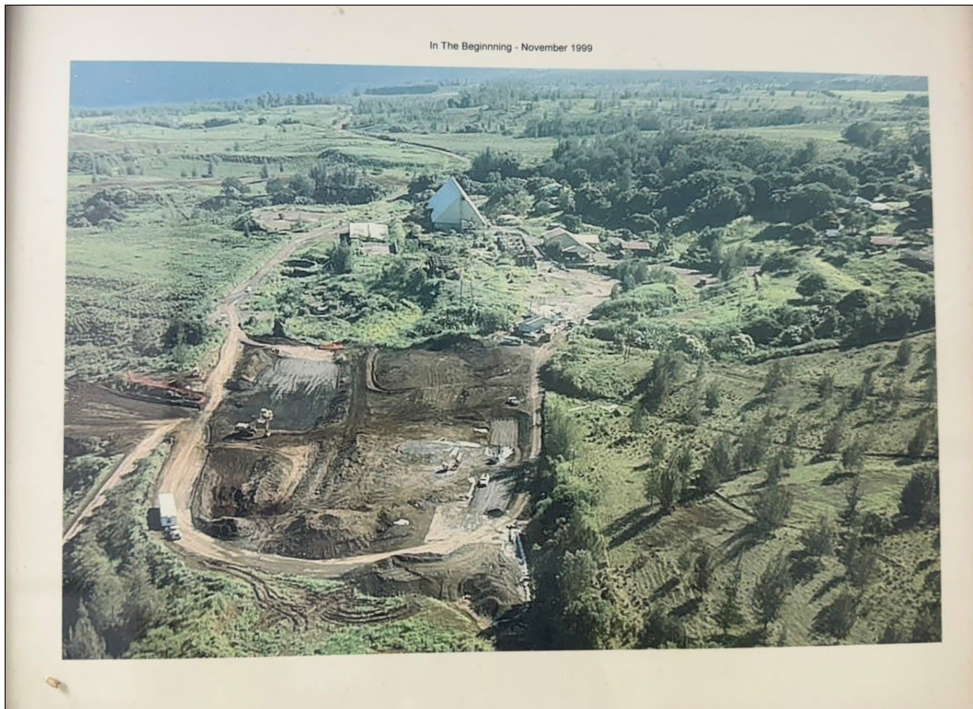
Figure 25. November 1999 photo on display at the existing Hamakua Energy Plant, showing the beginning of construction for the plant in 1999, note extensive ground disturbance; view to east
