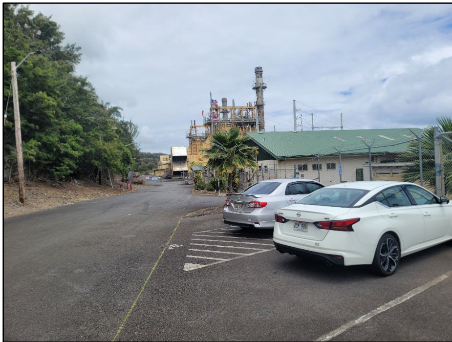
Figure 24. Photo of Kia Manu Street as it enters into the plant; view to west
