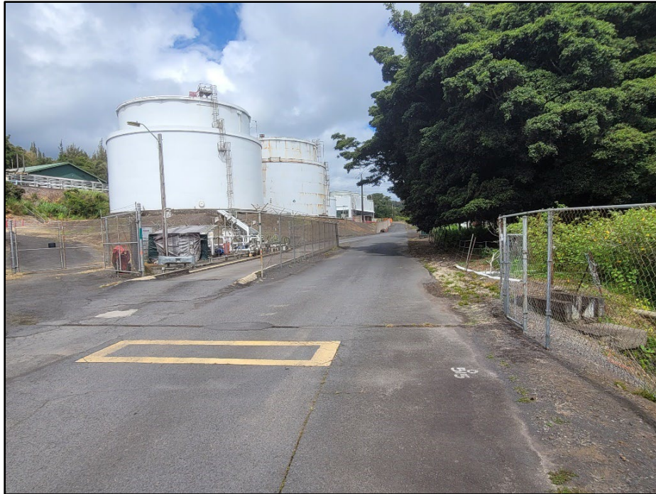
Figure 21. Photo overlooking Kia Manu Street at the plant entrance; view to west
