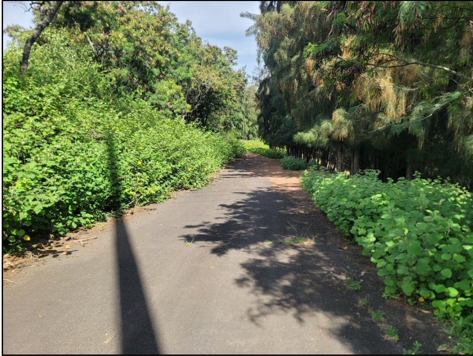
Figure 19. Photo of the paved driveway leading to the Haina Substation and proposed battery storage site; view to west
